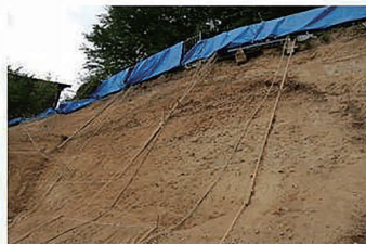
Geo-grid work sample: Kiyomizu-Dera, Kyoto
