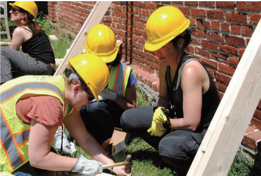
Fig. 2 Practicing emergency shoring techniques
