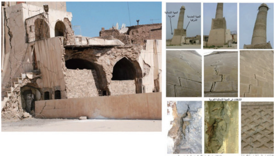
Fig. 5 The cracks in the base and the body of the minaret
