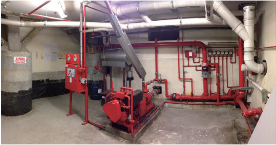
Fig. 8 Government Buildings - Sprinkler Pump and Control room
