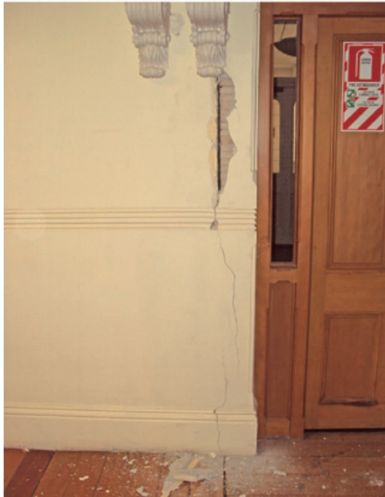
Fig. 7 Plaster damage from Earthquake 2013
